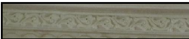
Fig. 13. P1a1 Decorative trim on roof
