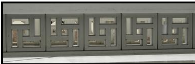
Fig. 12. P112 Decorative trim on wall
