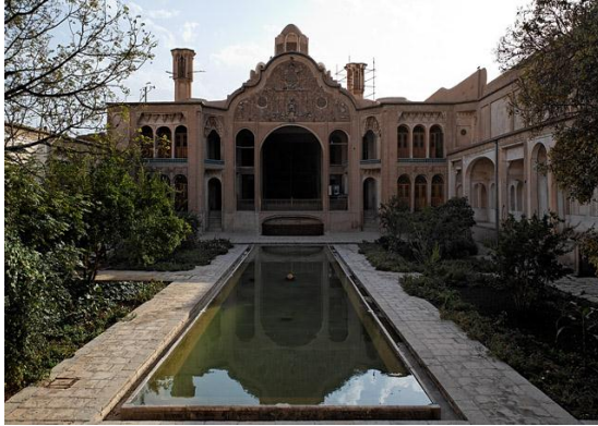
Picture No(4): Borujerdis house,Iran
